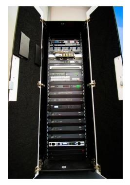
The Extron DVS 605 PiP unit is configured to allow any two of the listed sources to be displayed on the Custom Large Screen LED Video Wall. The images may be Picture in Picture (PiP), Pictures side by side (PaP).
